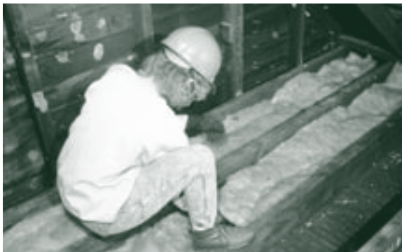
Energy efficiency improvements, such as the installation of insulation in residential buildings, helped America reduce its energy consumption after the energy crises of the 1970s.
