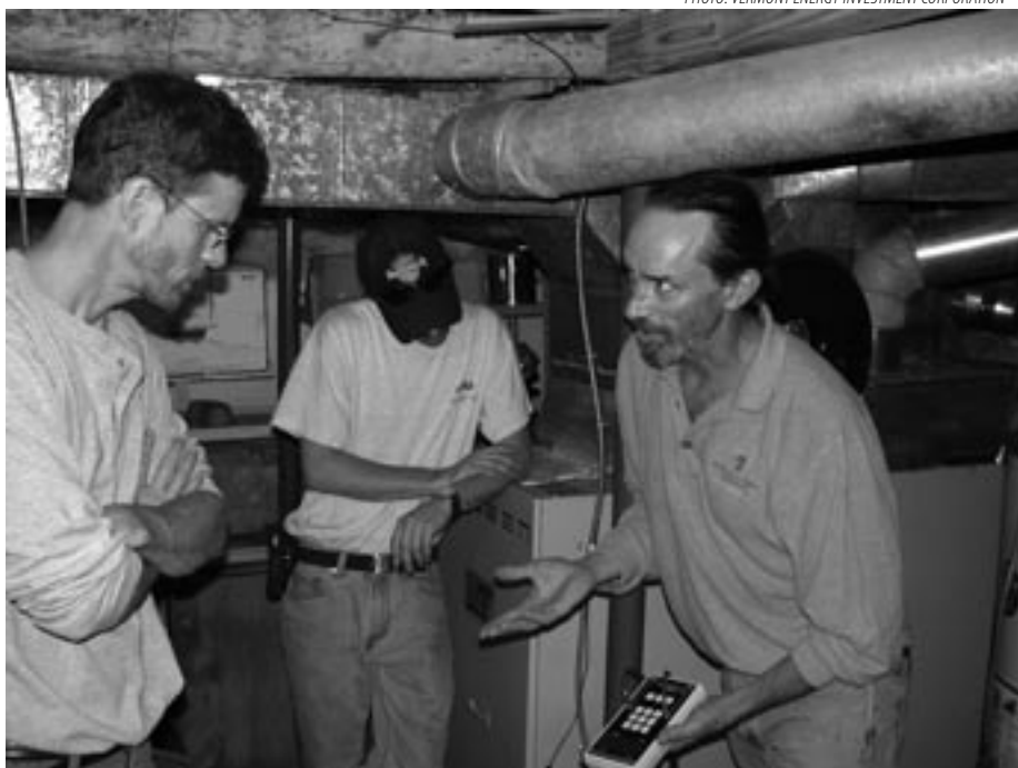
Contractors receive training on how to test and improve the efficiency of a heating system.
