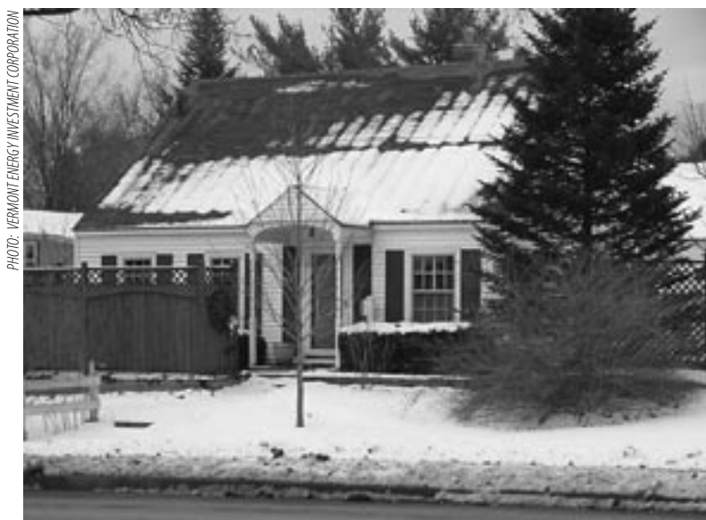
The snow has melted on the roof of this home in a pattern that shows the location of rafters and insulation below.
